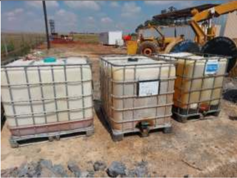
Photo 14. Diesel storage tanks placed on concrete hardstand
