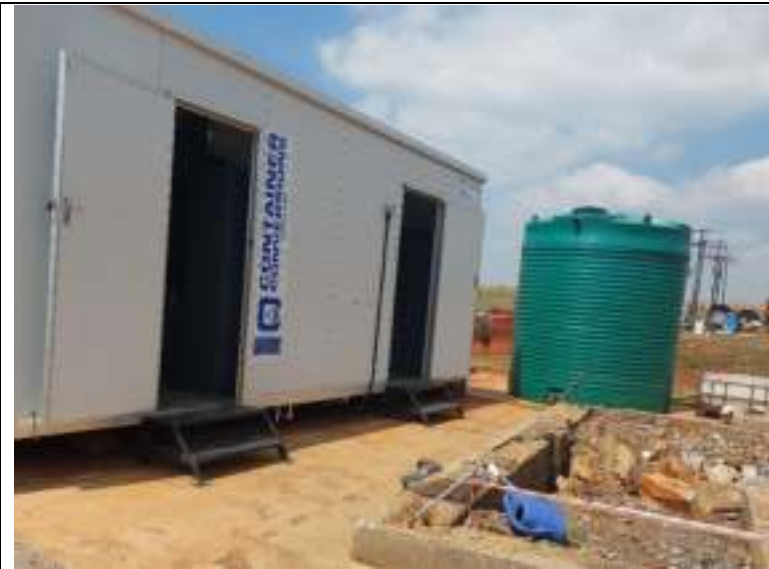
Photo 9. Containerised ablutions and potable water storage tank
