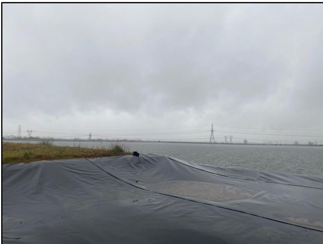
Figure 3. Lined spillway of RWD2 on the eastern side of the dam.
