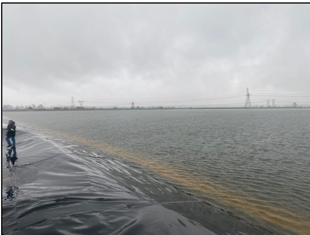
Figure 4. Freeboard of the RWD2 is sufficient; more than 0.8m.
